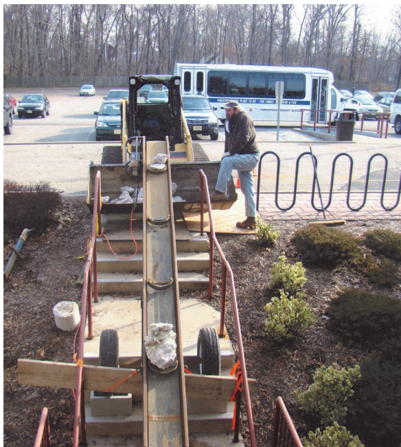
This machine carried concrete out of the lower level.
