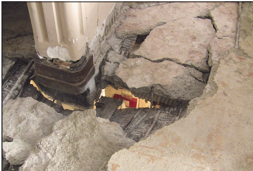
The underground explosion buckled the concrete floor enough to see through it.
